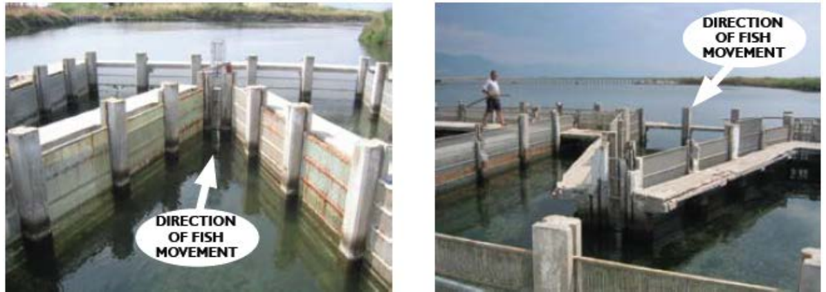
Figure 4.2. Permanent fish entrapment devices, which catch live fish as they move seawards (Vassova and Erateino Lagoons, Nestos Delta). The arrow shows the direction of fish movement (Source: E.T. Koutrakis).
